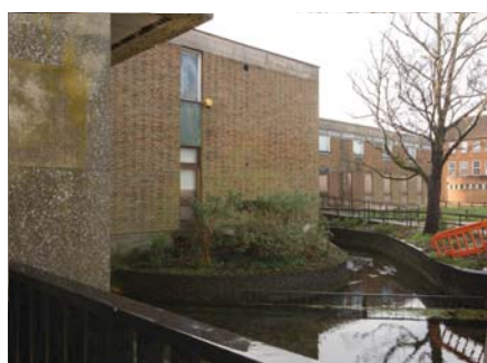
Purchase of Friarsgate medical centre for refurbishment
